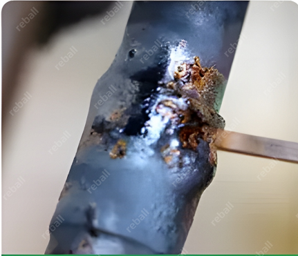
Iron surface welding
