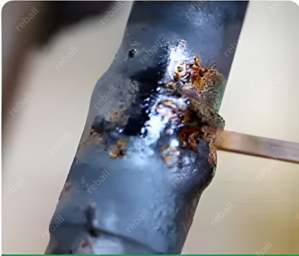
Iron surface welding
