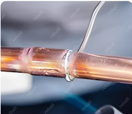
Copper surface welding
