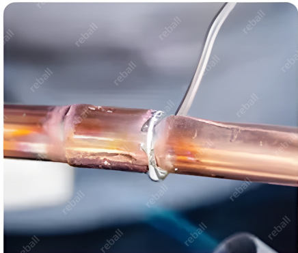
Copper surface welding
