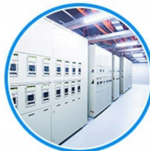
Industrial equipment testing
